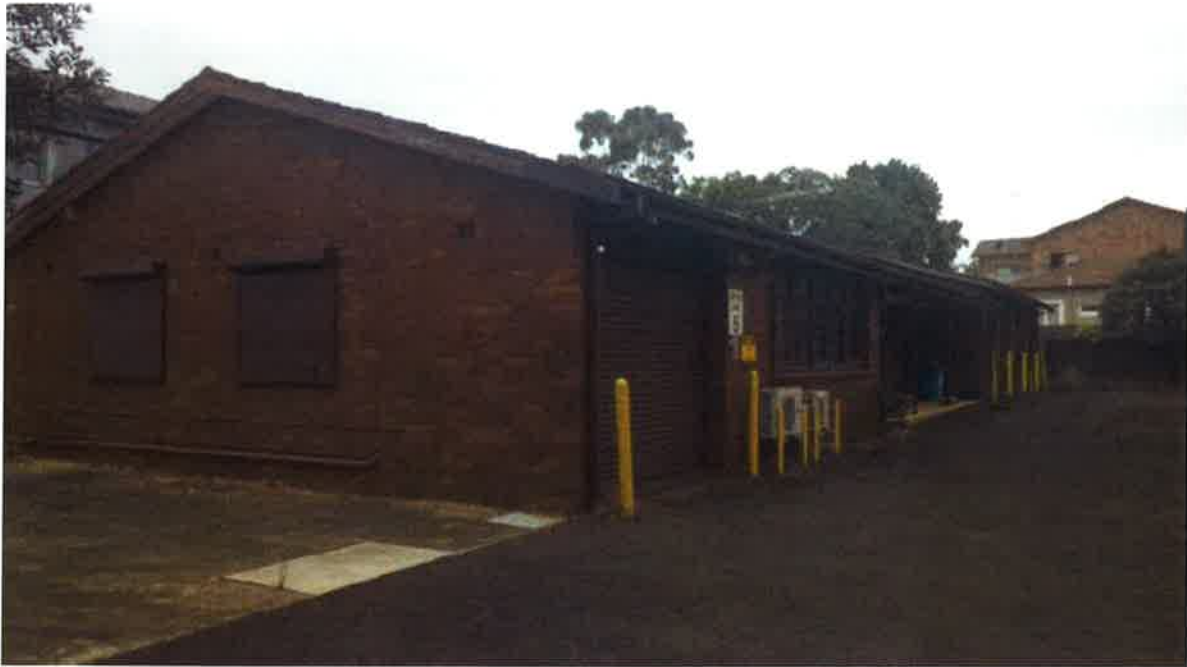
Figure 10: View of building (now demolished) at Lot 95 DP6743
