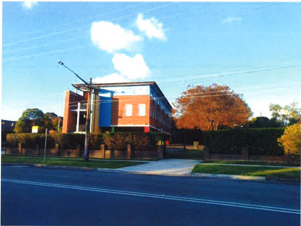
Figure 9: Image of current building at St Ambrose School
